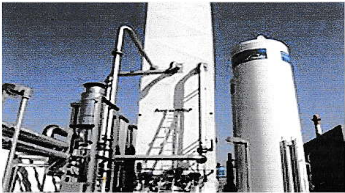
Nitrogen Cylinder, Liquid Nitrogen Distillation column in a cryogenic air separation plant
